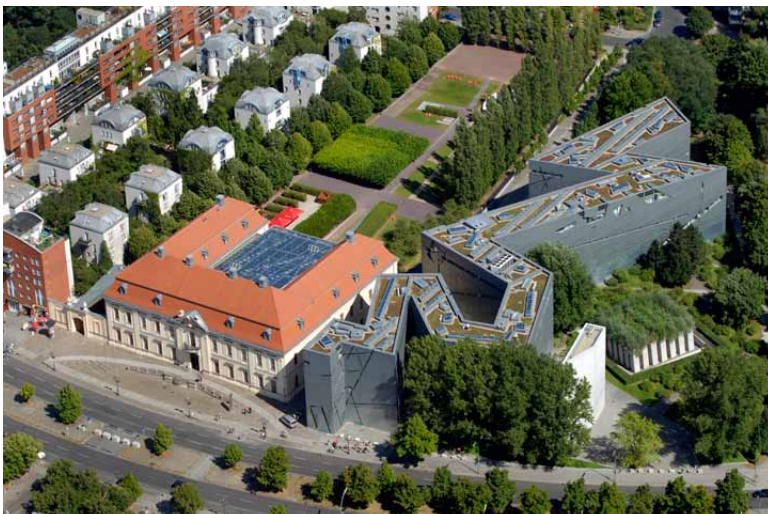
IMG. 01 – Aerial view © Guenter Schneider. Courtesy of D. Libeskind Stadium
