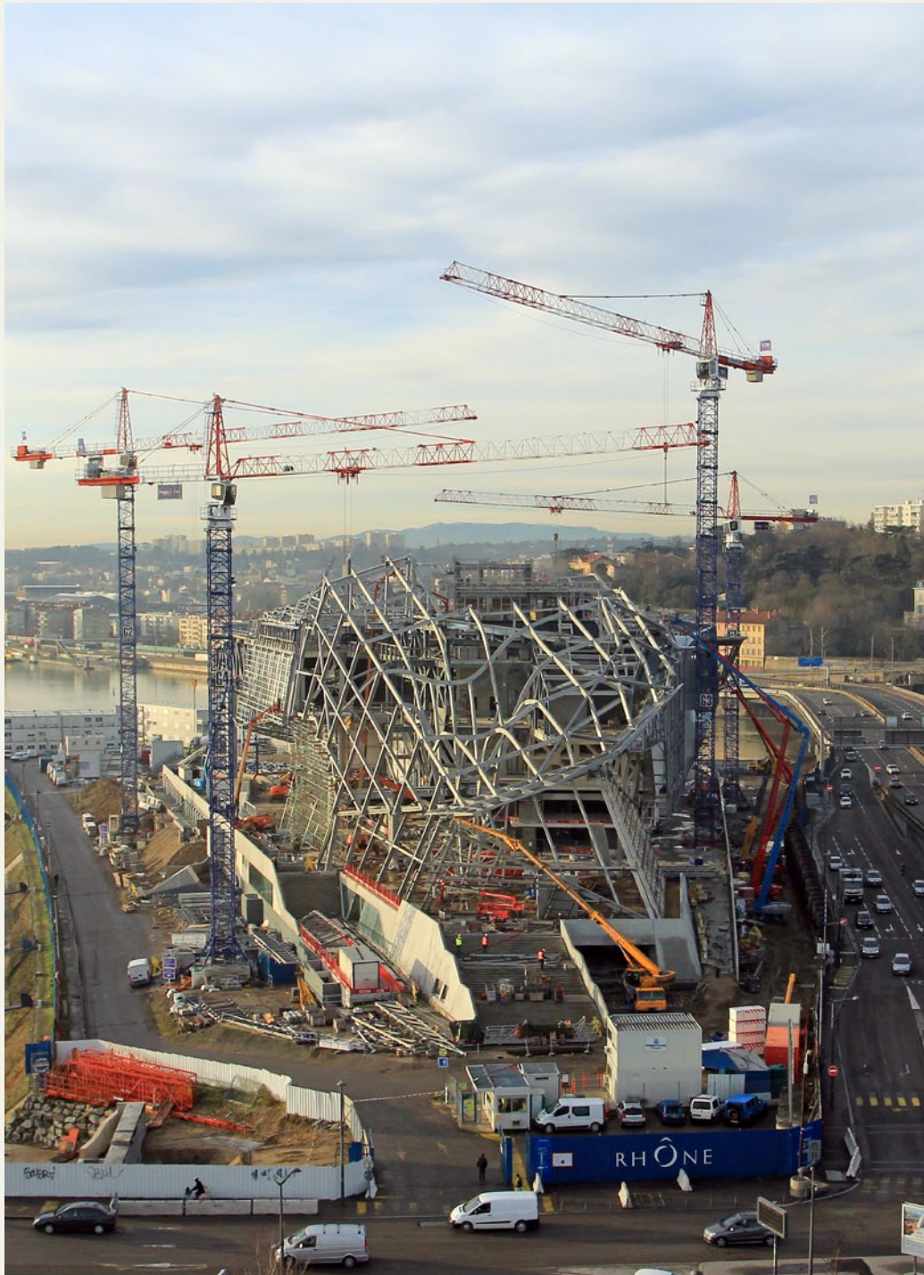
IMG. 2.27 — Musée des Confluences, Lyon, France. Project by Coop Himmelb(l)au. View of the construction site. © Hubert Canet, Balloide Photo.
