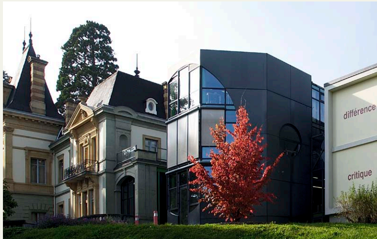
IMG. 3.29 — Exterior view of of the three buildings which compose the museum. © Musée d'ethnographie Neuchâtel. Photo by Alain Germond.
