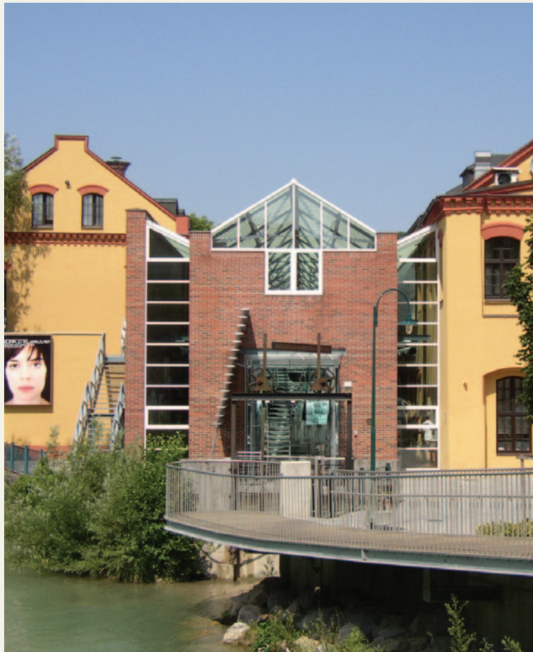
IMG. 1.24 — View of the entrance façade. © Walter Luttenberger.
