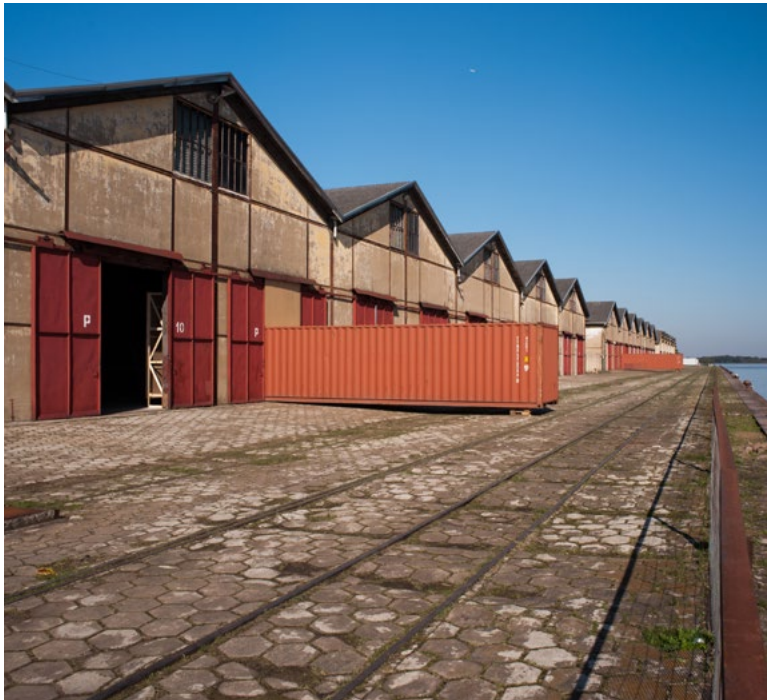
IMG. 01 — Warehouse spaces in Porto Alegre, by the Guaíba river (courtesy Fabio Del Re/VivaFoto)
